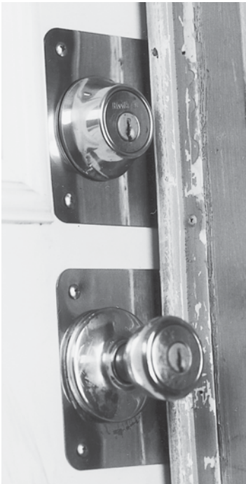
Figure 1.10 Typically key-in-knob locks for exterior doors are installed with a deadbolt.
