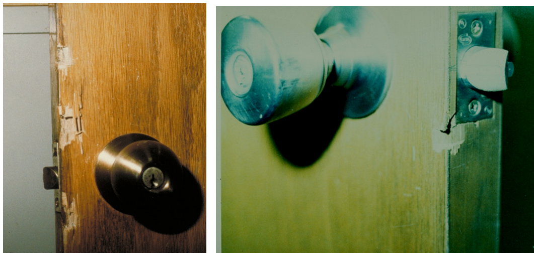
Figure LSS+3235 (ISP 16-3529 left, 17 right) Knob locks should not be used as the sole protection on exterior doors.
