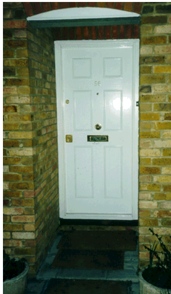
Figure LSS+3219 Recessed Left hand inward opening solid timber door with multipoint locking system, set in steel frame + additional top lock.
