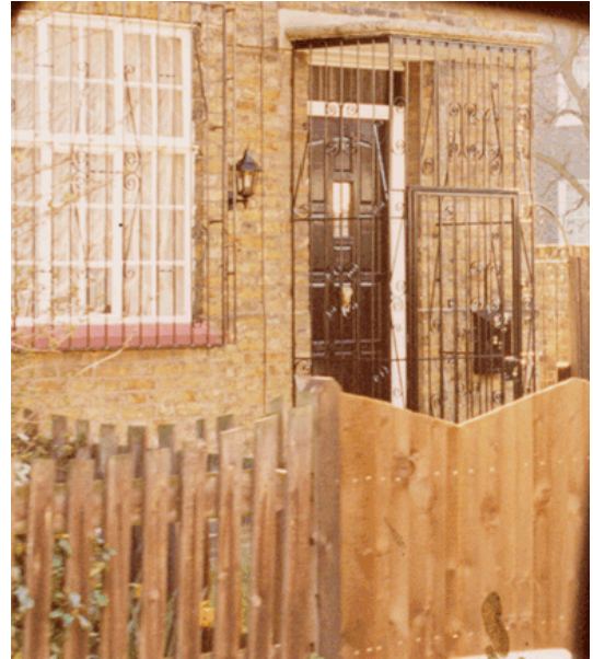
Figure LSS+3212 External - Steel cage protecting front door with right hand outward opening single lock with no cover plate. External steel grilles protecting windows; Internal - Inward opening solid timber door.
