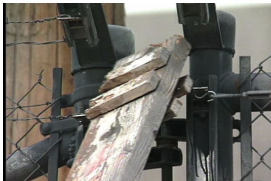
Figure LSS+4064 A climber is able to scale a fence by gaining a foothold. This is poor design.
