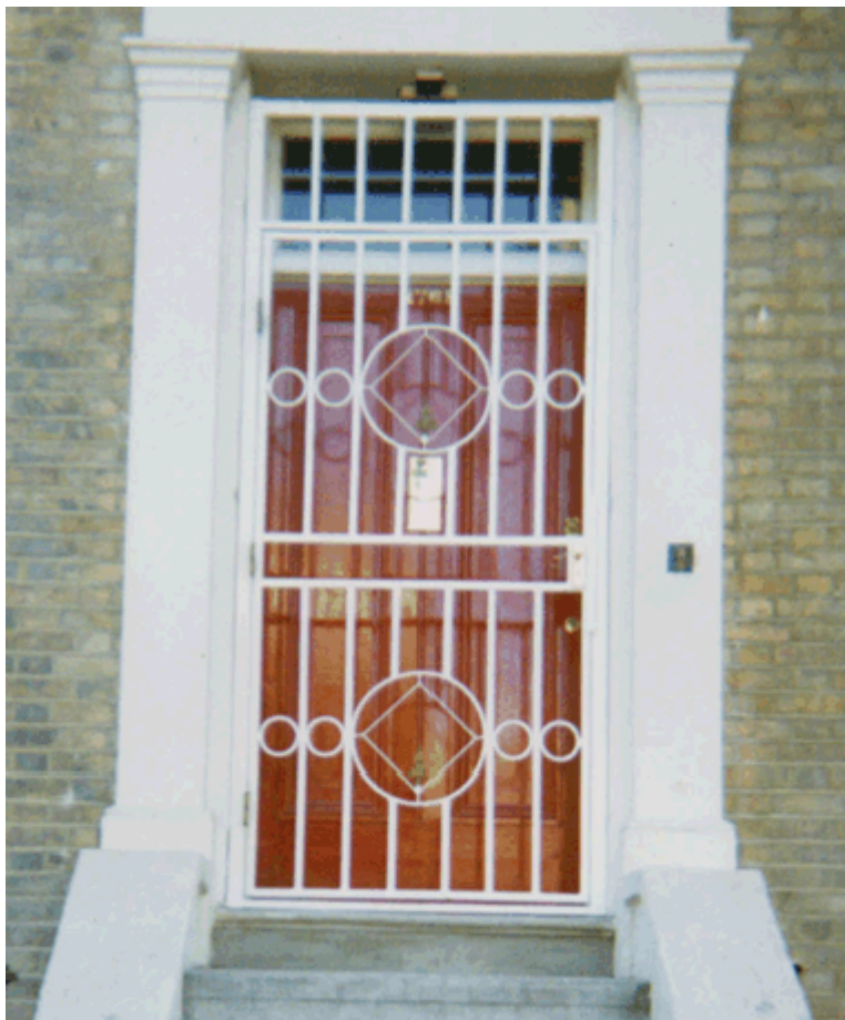
Figure LSS+3223 External - Recessed right hand outward opening steel gate with three standard butt hinges and no cover strip; Internal - Right hand inward opening timber paneled door with two locks visible.
