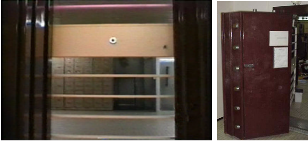
The Lips vault door and barrier gate into the strong room.
