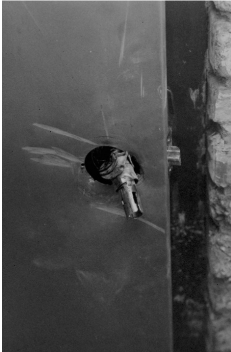
Figure LSS+3239 (ISP 18-3529 left, 20 center, 21 right). A pipe wrench can be utilized to twist loose a key-in-knob or cylinder lock.
