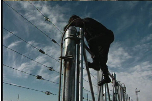
Figure LSS+4064 A climber is able to scale a fence by gaining a foothold. This is poor design.
