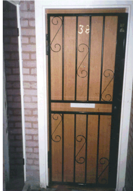
Figure LSS+3216 External - Right hand opening steel gate with single lock, full cover plate and rising butt hinges;
