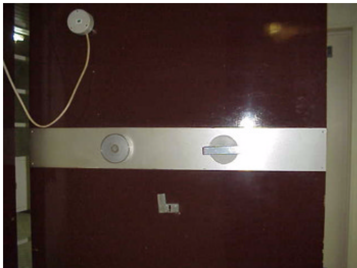
Lips safe door, showing combination lock (left), bolt actuating handle (right) and lever lock (center)
