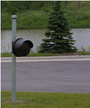
Figure LSS+4059 A monostatic system radiates a coverage pattern much like a flashlight beam. The dark gray area shows diminished coverage. Courtesy of DOE Office of Security and Safety Performance Assurance.
