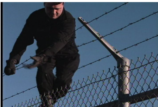
Figure LSS+4065 Intruders are able to penetrate a facility using a variety of techniques. Materials are removed from the fence and used as an aid to the climbing process. The top of the fence line can be used for support. A
