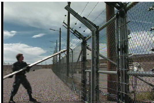
Figure LSS+4064 A climber is able to scale a fence by gaining a foothold. This is poor design.
