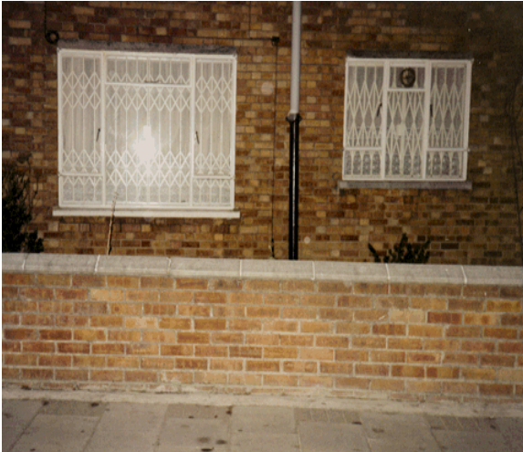
Figure LSS+3209 Internal concertina mild steel window grilles (Center locking) behind 6 mm float glass casement window.
