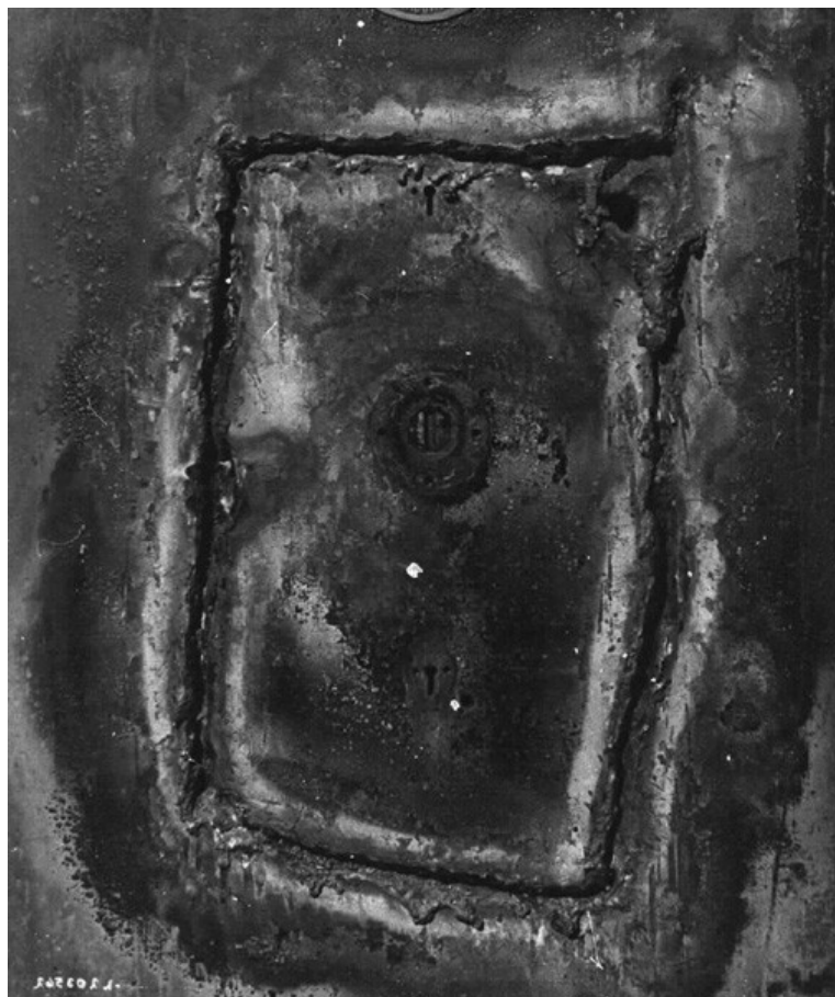
Figure LSS+3523 Additional examples of the use of a torch. In the photographs, the lock box is burned out.
