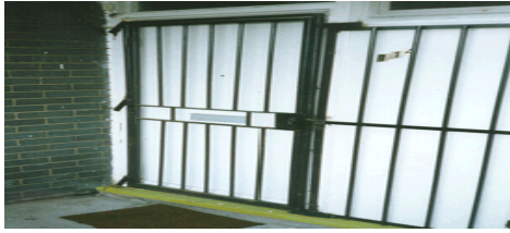
Figure LSS+3217 External - Right hand outward opening steel gate, single lock, no cover plate and standard butt hinges; Internal - Right hand inward opening solid timber door, one lock visible.
