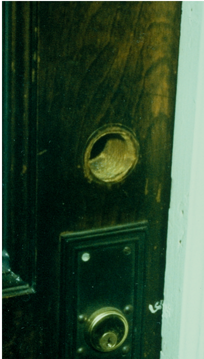
Figure LSS+3237 (ISP 26-3529 left, 27 right). Cylinders can be pried loose if not mounted properly.
