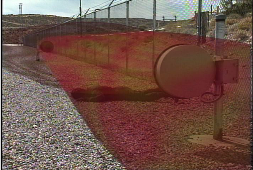
Figure LSS+4059 A monostatic system radiates a coverage pattern much like a flashlight beam. The dark gray area shows diminished coverage. Courtesy of DOE Office of Security and Safety Performance Assurance.
