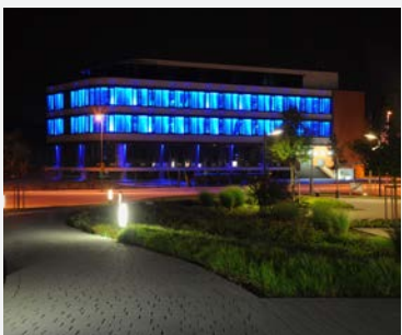
Elbe Office, Germany
