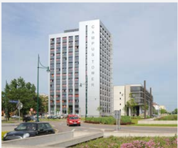
Magdeburg Campus Tower, Germany
