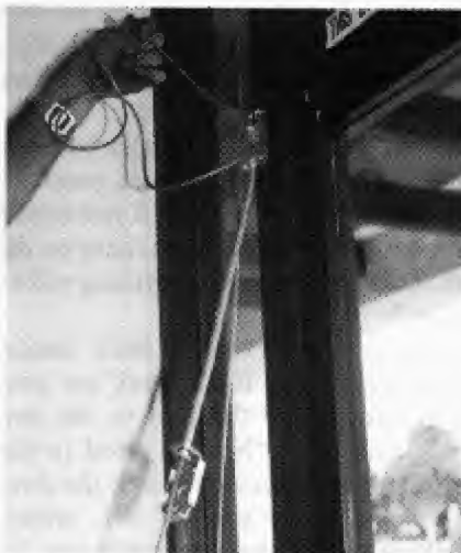
6. Proper method for feeding the armored door cord into the door.
