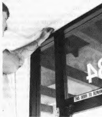
4. Coaxing the wire through the hollow door frame.
