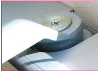
13 A flat screw holds the arm to the pinion.
