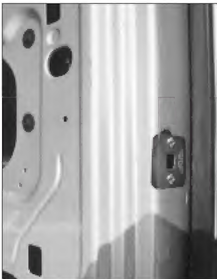
Photograph 5. Door jamb trimplate.
