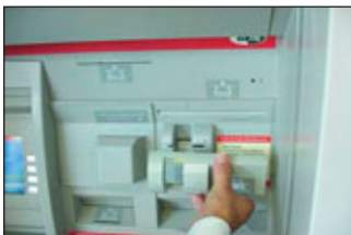
1. Equipment being installed over existing bank card slot.
