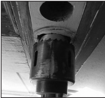
13. The guide is pushed into the hole saw when cutting.
