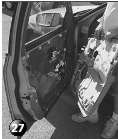
27 Plastic clips hold the door panel in place, and it may need a little coaxing. Be careful not to break the clips or the clip holders
