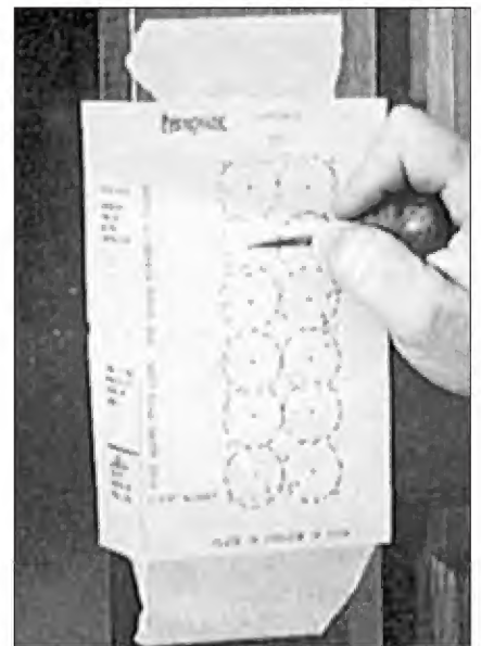
5. The end result must be a rectangular cut out of 5-3/8" high and 1-7/8" wide.
