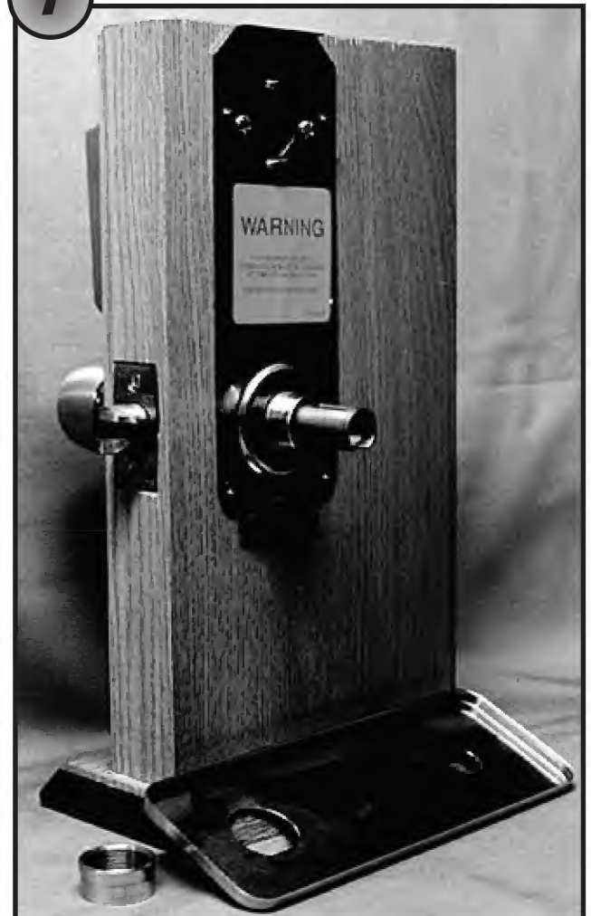
The standard unified trim plate and threaded ring is next to install.
