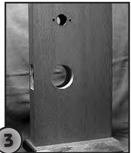
3 The lock mount with the three additional holes required for installing the Unican® 1000 lockset.
