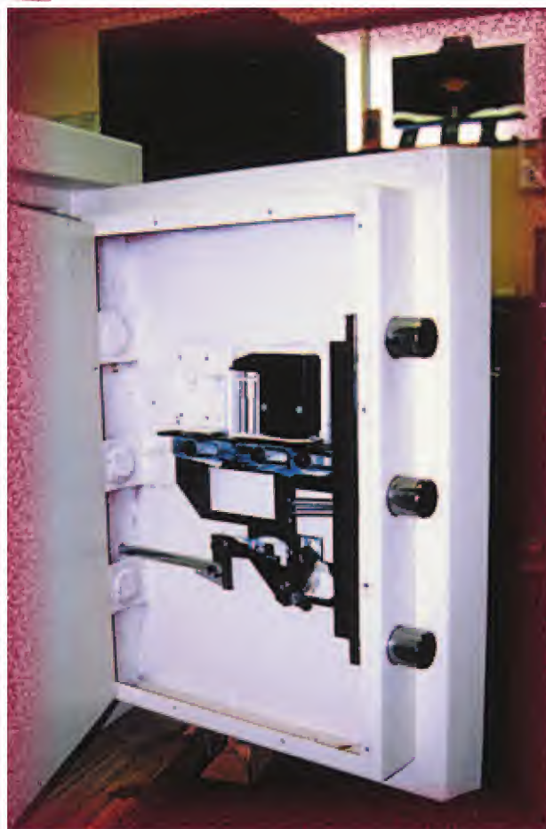
5. Full view of TL-15 door, three moving bolts and detent mechanism.
