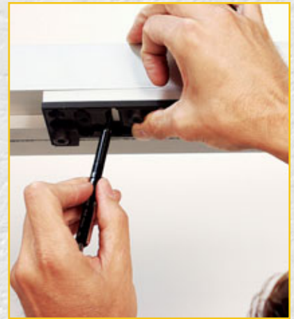
5. Locate the two slots and mark.
