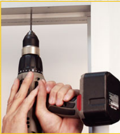
3. Mark and drill the door frame.
