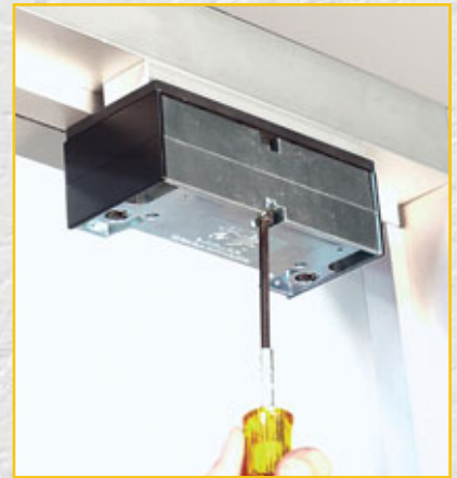
11. Attach the MS Maglock to the mounting plate.
