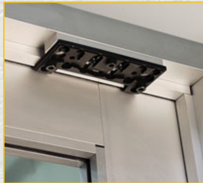
7. Attach the MS Maglock mounting plate with the provided bolts.
