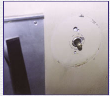
6. Note tube around dial spindle to keep insulation away from dial spindle.
