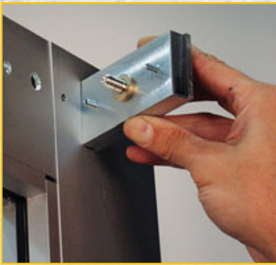
9. Locate the armature onto the door.
