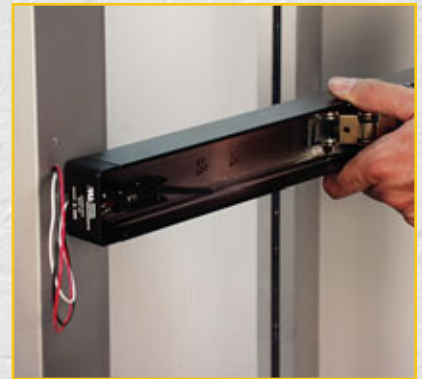
14. The 8099 Pushbar/Switch device fastened to the door.
