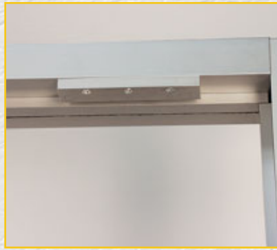
4. Secure the filler plate to the frame.
