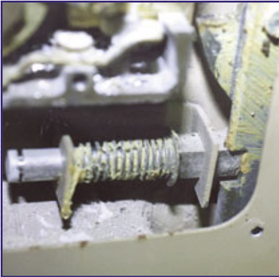
8. Close up of the fired relocker fitting into cut out on vertical bolt bar.
