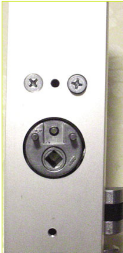
8. The view from the inside door surface.
