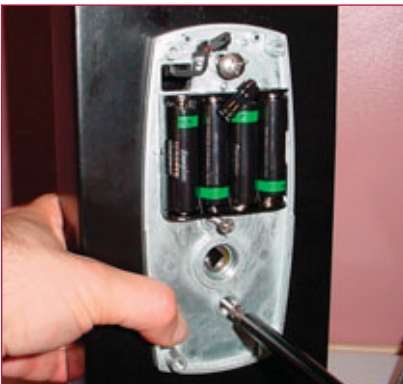
12. Three screws will attach the inner assembly.
