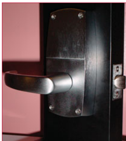
16. The inside handle should always retract the latch.
