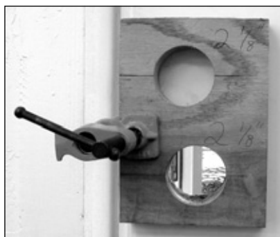
2. Like many non-commercial doors, this one needed to have the 2-1/8" cross bore relocated from 2-3/8" to 2-3/4".
