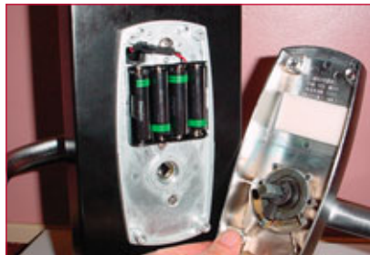
14. Insert the matching spindle into the hole in the inside escutcheon.
