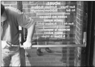
18. Finishing up the panic device.
