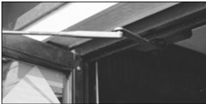
19. Install and attach new closer.
