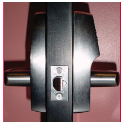
17. The completely installed lock.
