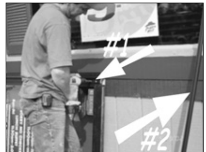
7. Securing hinge with self-drilling screws.
