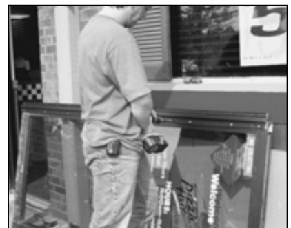
8. Drilling through holes for sex bolts.
