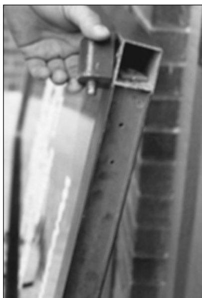
6. Removing top pivot.
