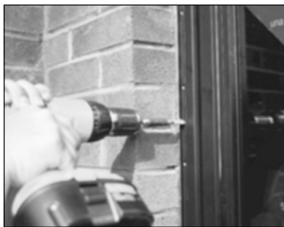
12. Driving self-drilling screws.
