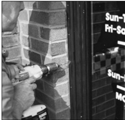
11. Drilling pilot holes.
