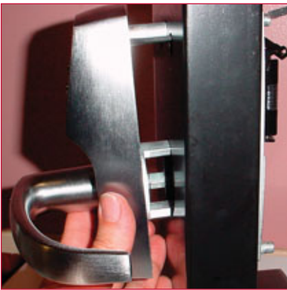
11. The outside assembly is ready to install.
