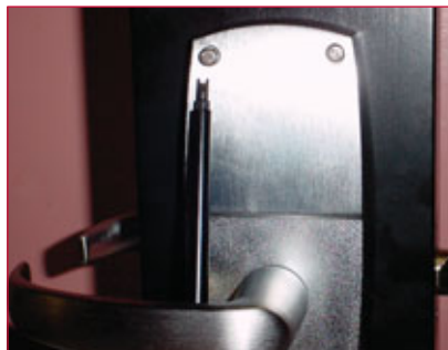
15. Fasten with four security (spanner) screws.
