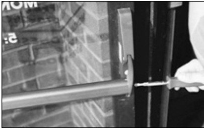
17. Attaching push bar to hinge side of door.
