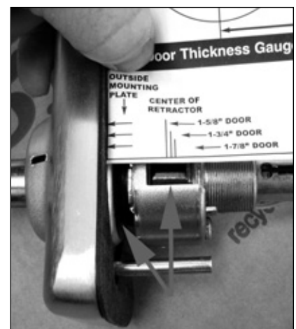
3. The door thickness of this door is 1 3/4". The lockset can accommodate anything from 1-5/8" to 1-7/8".
