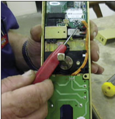
22. Lock battery case installed. Wire harness in place. Wire plug and wire need to be clear of motor in case of overheating and causing melted wire.
