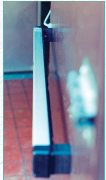
26. The panic device on the door is Securitron's TSB. (Touch Sense Bar.) This bar is used in conjunction with a Maglock and, in this case, a DK-26. The TSB operates by recognizing a touch (even through light clothing) and releases the Maglock, permitting egress from the building. This unit was installed on the kitchen door of a restaurant.
