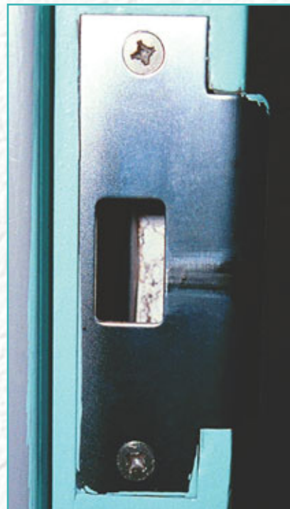
29. This, of course is the standard ANSI strike for the L1000.
