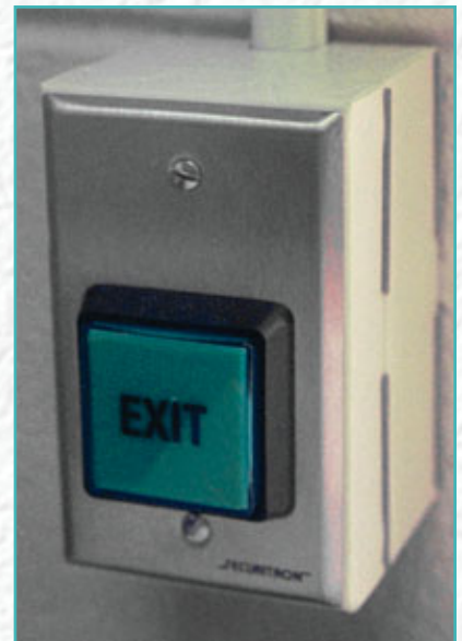
9. This is a second SEPB2 that was located just to the right of the church secretary's desk to allow the secretary to admit people that did not have the combination to the touch pad.
