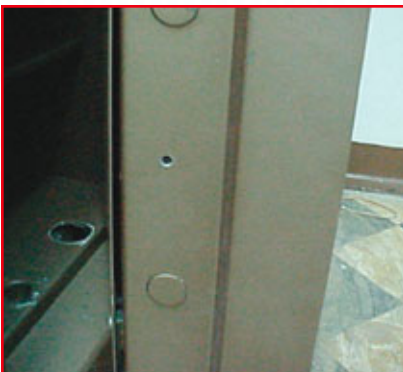
9. The hole drilled in the edge of the door.
