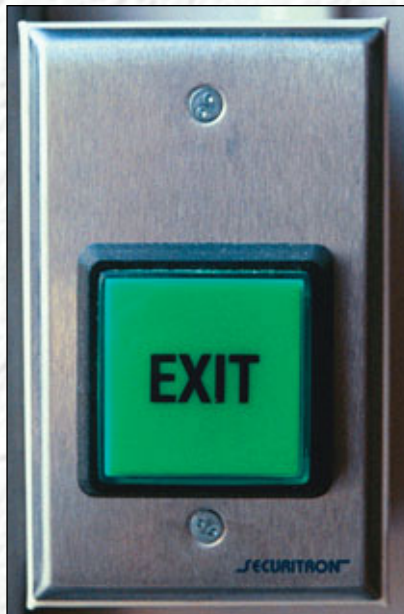
8. The Securitron request to exit switch (SEPB2) is mounted to the Wire Mold junction box and allows for free egress from the church by the people that did not have the combination to the touch pad.
