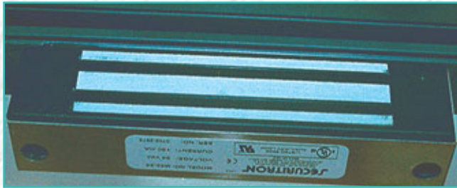
20. The Model 32 magnet mounted to the bottom of the header rail on a storefront door. Securitron provides all the necessary mounting hardware needed
