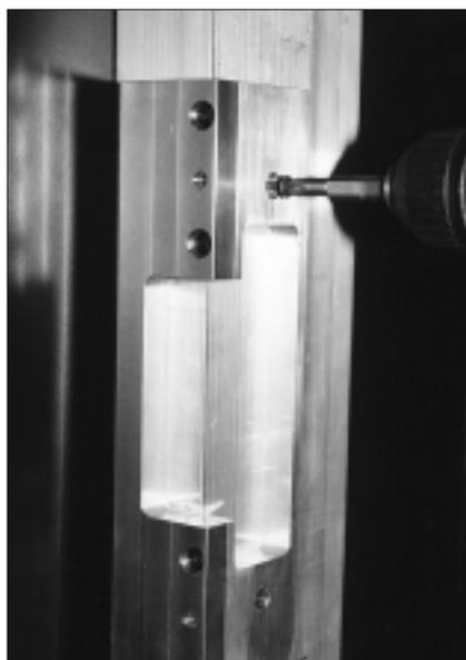
10. Use the self drilling drywall screws to attach the template to the frame.
