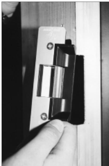
12. After checking for the initial fit, the U-Tabs were installed and the strike mounted to the frame.
