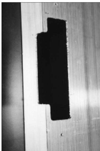
11. The finished cut includes holes for attaching the U-Tabs needed for mounting the electric strike.
