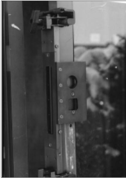
5. After removing the existing push bar and pull handle, the HIT-45 is clamped to the door and ready for cutting.
