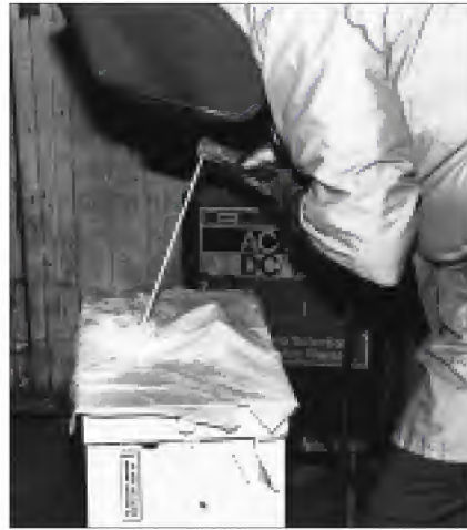
15. Repairs must be done with electric welding.
