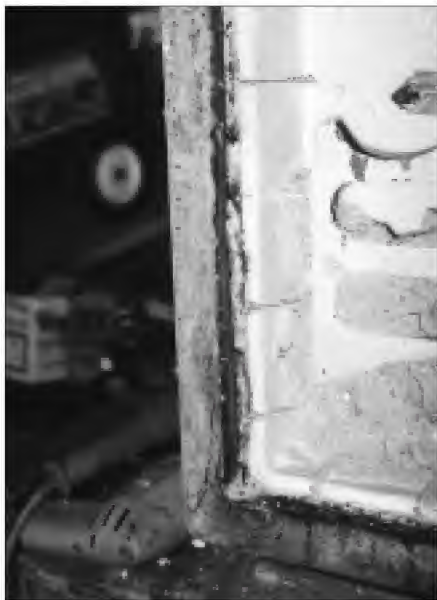
12. Opening side of safe door with insulation removed to show melted edge of door and the interior metal laminate.
