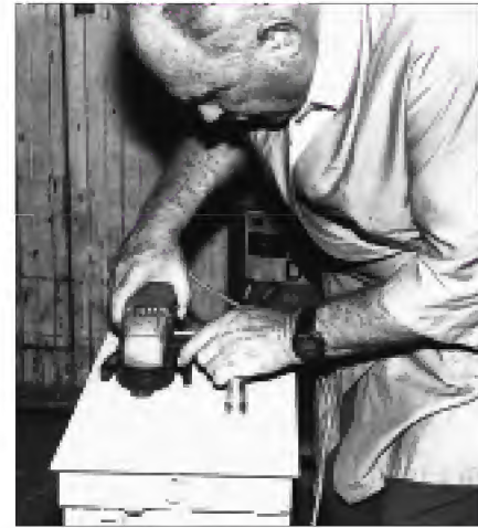
16. Grind the repair area smooth and putty before painting.
