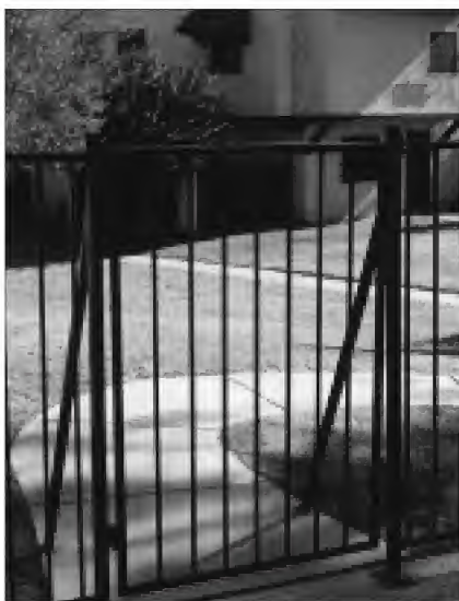
3. Maintenance gates also must be locked and swing shut automatically.
