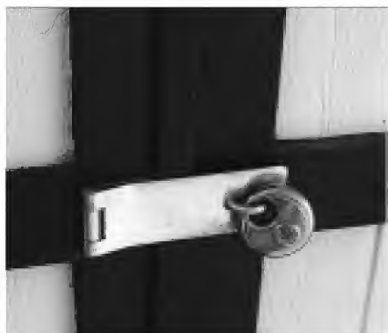
4. This large hasp and round padlock were used to protect this shed.
