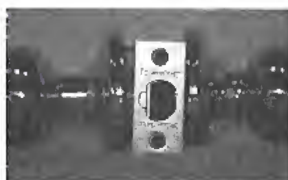
1. The Master knobset can be identified by its name on the latch faceplate...
