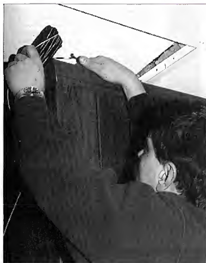
8. Running the wire above the ceiling and down through the wall.
