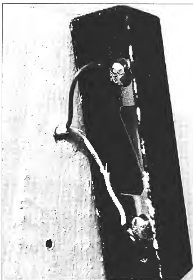
4. After disconnecting the doorbell transformer, remove the doorbell switch.
