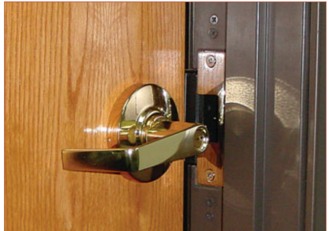
4. Steel doors and frames.
