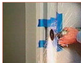
8. Cutout the required section.
