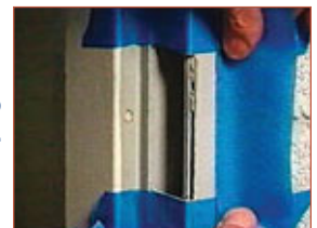
7. Use masking tape to protect the jamb.
