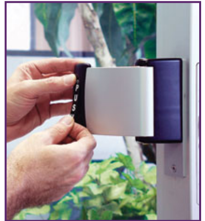
15. Attach the supplied "PUSH" or "PULL" sticker to the outside end of the paddle. Paddles are ordered handed, but can be switched in the field. The installation instructions show how this can be simply achieved.
