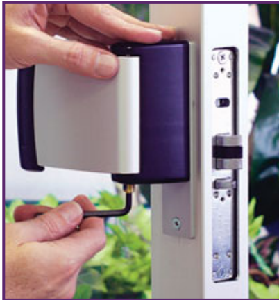
13. Tighten a setscrew on the bottom of the paddle to retain the pivot pin with an Allen wrench.
