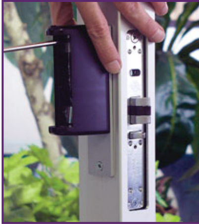
11. Secure the paddle escutcheon to the adapter plate with the supplied #10-32 x 1" screw in the top binder post and the #10-32 x 1-1/2" screw in the lower mounting hole of the escutcheon.
