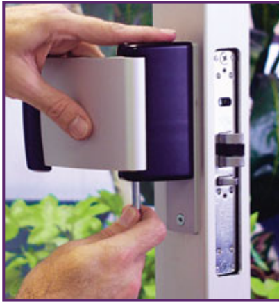
12. With the paddle positioned in the escutcheon, insert the pivot pin.
