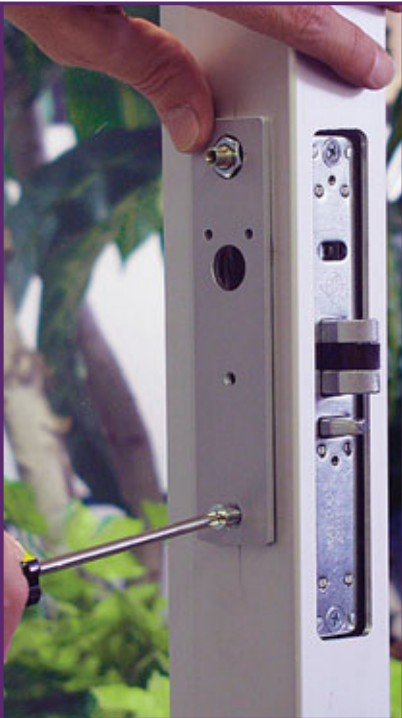
10. For this retrofit, you will need to install the 91-0912 adapter plate first. This new product covers the previous cutout for the exit indicator and gives a clean, finished look to the installation. Fit the adaptor plate over the binder post on top and secure it with one flat head screw on the bottom.
