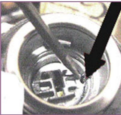
17. By drilling at this location you will be providing an access hole for the sidebar pressure tool.
