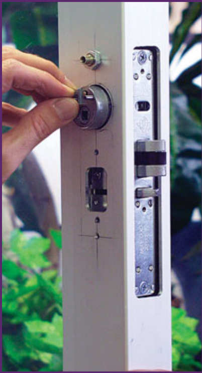
9. Install the cam plug supplied with the paddle in the deadlatch.
