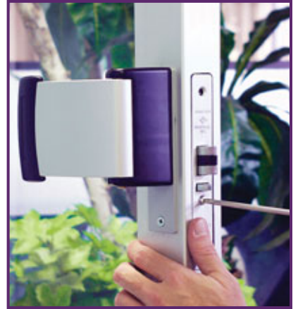
14. After checking the operation of the paddle, install the deadlatch faceplate.
