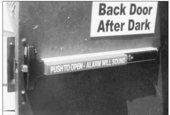
12. The completed assembly.
