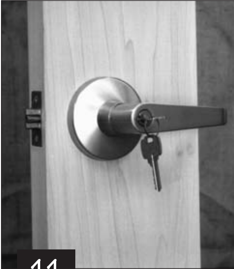
Completed installation showing outside lever.
