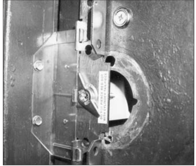
5. The V40's back plate slid over the mounting tabs.
