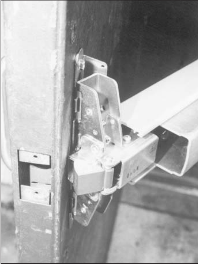
6. The tabs slide easily into the holes on the back plate.
