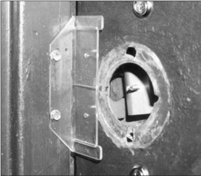
4. Plastic strike mounting template.
