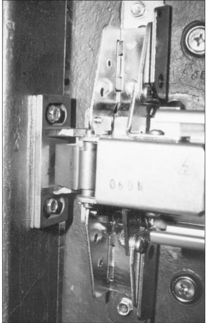
8. The detail of the 99 Strike and V40 back plate.
